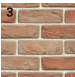
Light brown brick Light grey mortar
