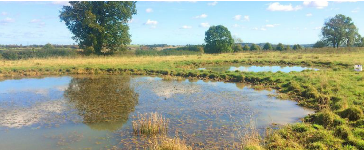
Figure 7-1 - Planted detention basins as part of the route
