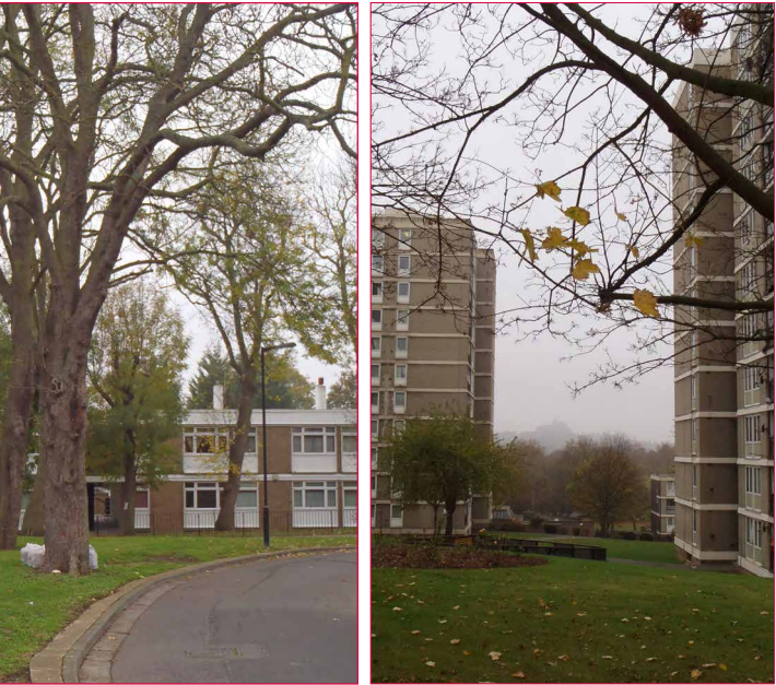
Torridge Gardens, 60s development with modern terraces and a block of flats set in open space
