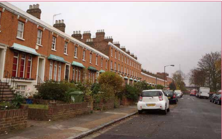
Historic Regency terrace
