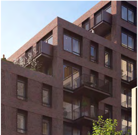
Example of screen for Wind Mitigation: Solid side panel to standard height
