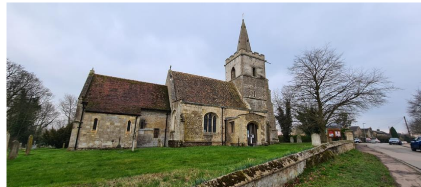
Figure 9-3 – Grade I listed Church of St Peter
