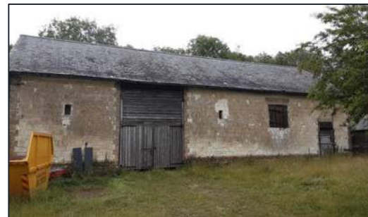
Fig.4.5.1. A bank barn construction of stone with large barn door and hay loft on the eastern elevation. A number of vents present on each elevation but all with intact grills. One of the farm workers informed the surveyors that barn owls have roosted within the building but not recently.
