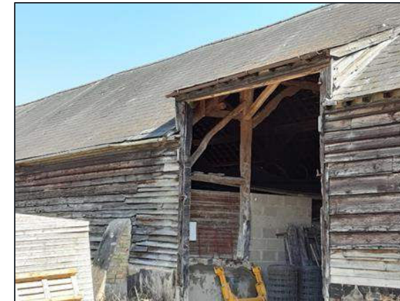
Fig.4.5.1. The barn has been totally re-roofed with slate since 2020, with mortise and tenon A-frame construction suggesting pre-18th century construction. Evidence of habitation by barn owl with streaking on beams (age not determined).
