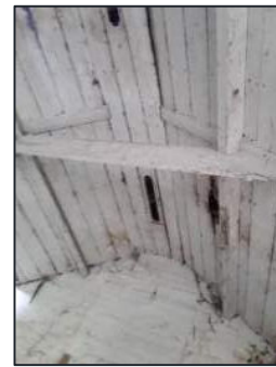
Fig.4.2.2 The resident barn owls using the roof void of the old milking parlour with the resident male barn owl exiting the vent shown in the barn during the survey in 2022.
