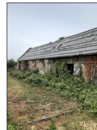
Fig.4.1.1 Netherhall Farm is an 18 th century farmstead property with a main farmhouse (Netherhall Grange), converted stable block (the Cart Lodge) and series of out buildings. The Farmhouse and stables represent little opportunity for barn owls. However, the existing stables and barn are a confirmed breeding site for barn owl and act as an ARS during the non-breeding season.
