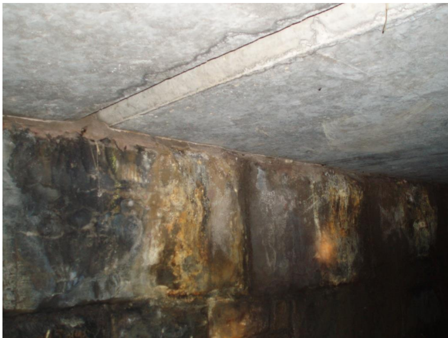
Fig 2, Tunnel at approximately 160m from the Diggle Portal
