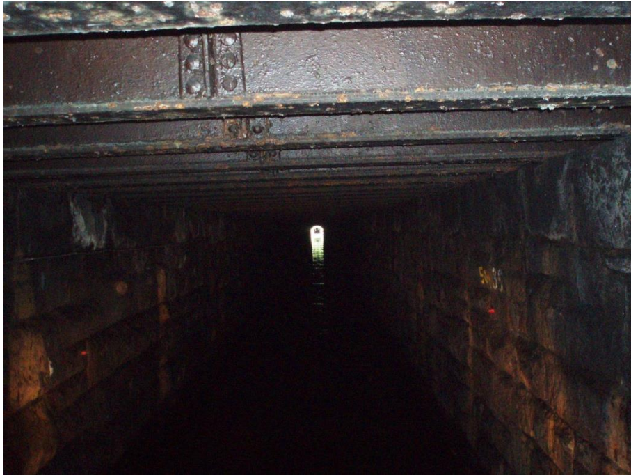
Fig. 1 Tunnel at approximately 130m from the Diggle Portal
