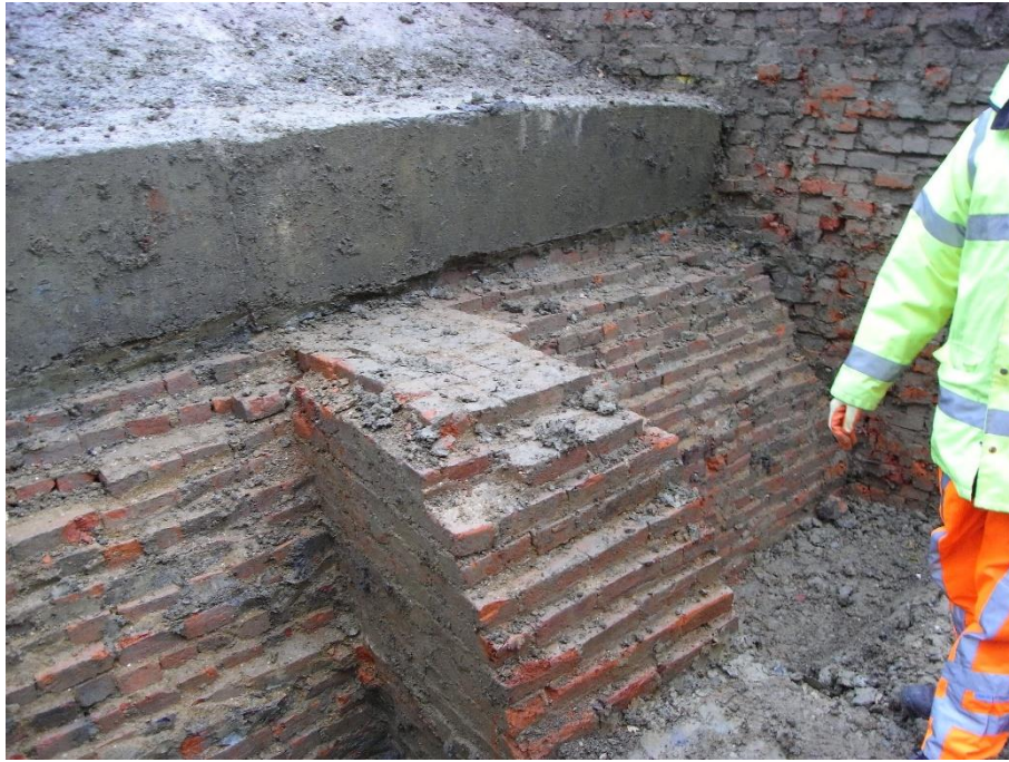
Fig. 5 Photograph of haunching at a canal arch bridge
