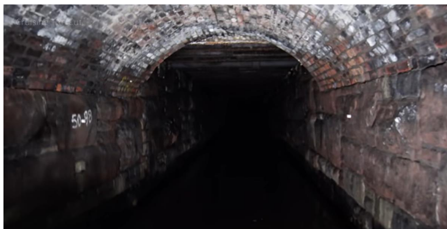
Fig. 3 Tunnel at approximately 100m from the Diggle Portal looking towards the flat deck 2
