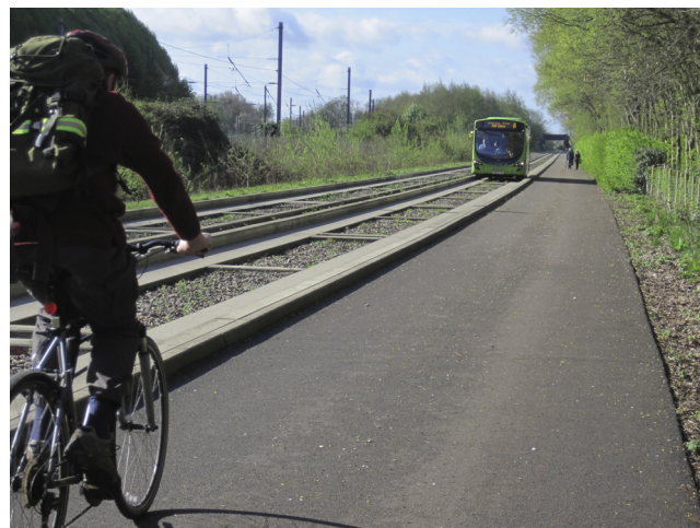
Fig. 1. The Cambridgeshire guided busway
