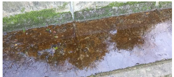
Figure TR5.1.A-14 – Concrete Channel 2
