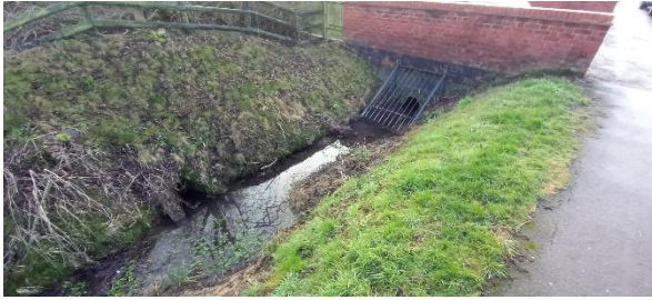
Figure TR5.1.A-49 – Grated Culvert
