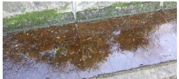
Figure TR5.1.A-12 – Concrete Channel 2
