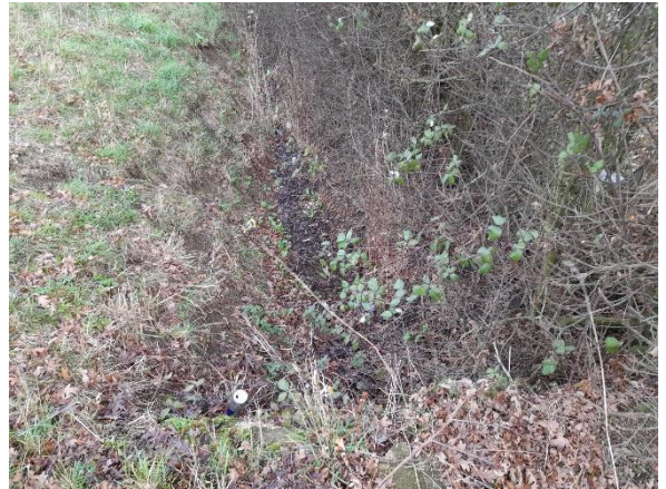
Figure TR5.1.A-74 – Dry Ditch
