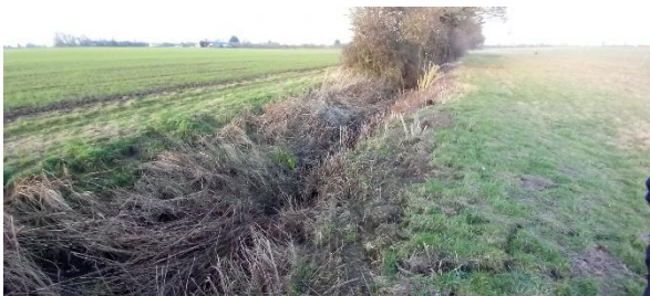
Figure TR5.1.A-71 – Vegetated Drain
