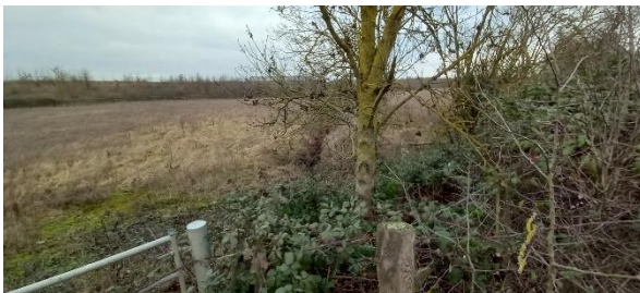
Figure TR5.1.A-53 – No access through gate
