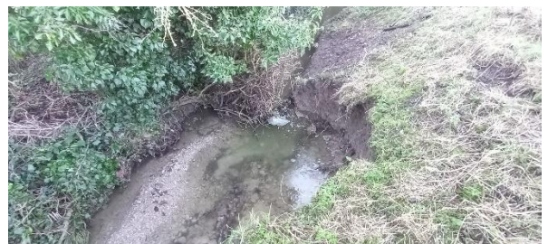
Figure TR5.1.A-6 – Bank Erosion
