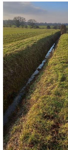
Figure TR5.1.A-70 – Drain Overview
